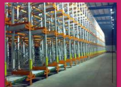
Shuttle Pallet Racking
