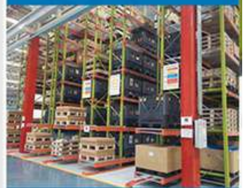
Very Narrow Aisle Pallet Racking System
